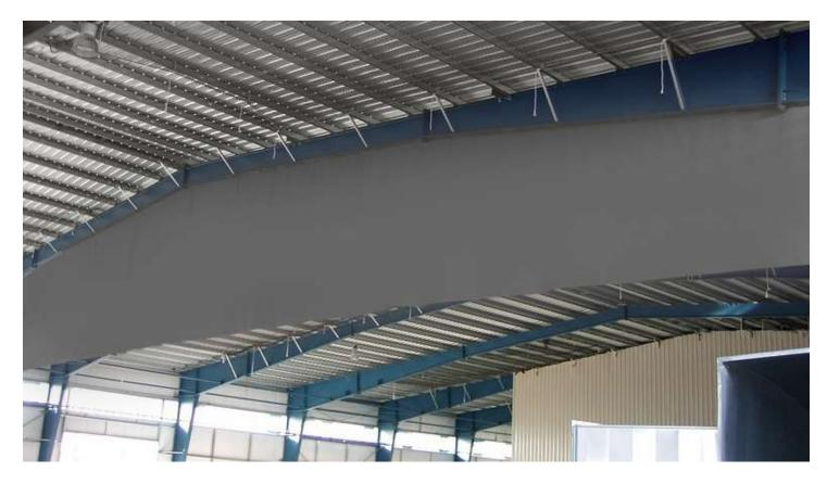
Aeroduct Draft Curtains are an effective solution designed to provide protection against smoke spread in commercial and industrial structures. Secured to structured steel, draft curtains ensure smoke and hot gases arising from the fire to be channelized to exchaust and extracting point.
