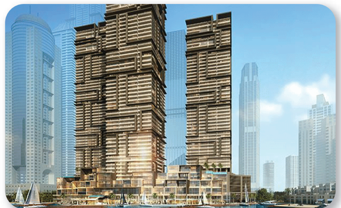
MARINA GATE TOWER, DUBAI - UAE
